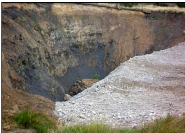
Figure 21. Backfilling the sinkhole in 2014, when the Bowland Shale mudrocks were exposed on the left side (photo: PDNPA).
