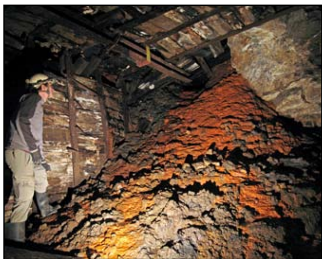
Figure 19. A run-in of mud and debris where a high-level cross-cut within an early phase of the mine had encountered even older workings left by the 'old man' (photo: Rob Eavis).
