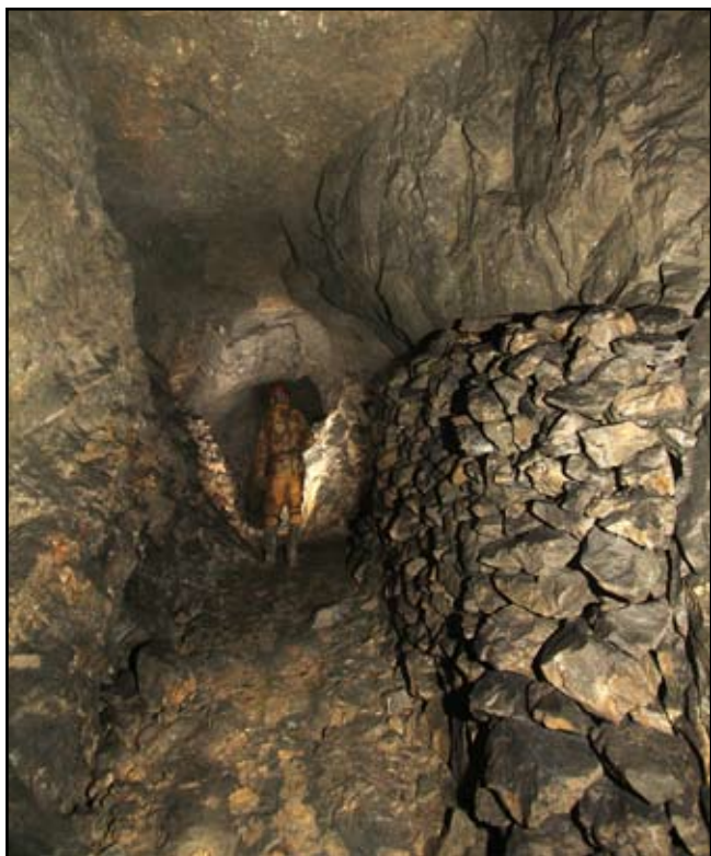
Figure 11. Typical gallery, with stacked 'deads' left by the 'old man' in the upper parts of the vein (photo: Rob Eavis).
