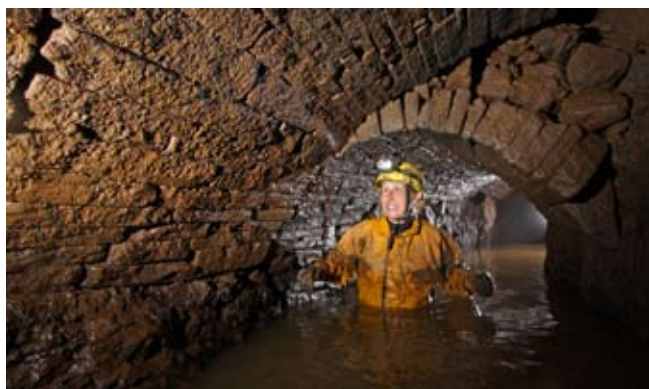
Figure 12. Stone arching that supports the roof in Morewood Sough, west of Stoney Middleton (photo: Rob Eavis).
