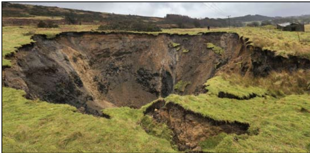
Figure 17. The sinkhole that developed over the chimney collapse in December 2013 (photo: The Independent).
